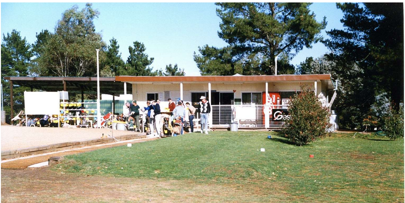
IMAGE H2 – the original clubhouse
