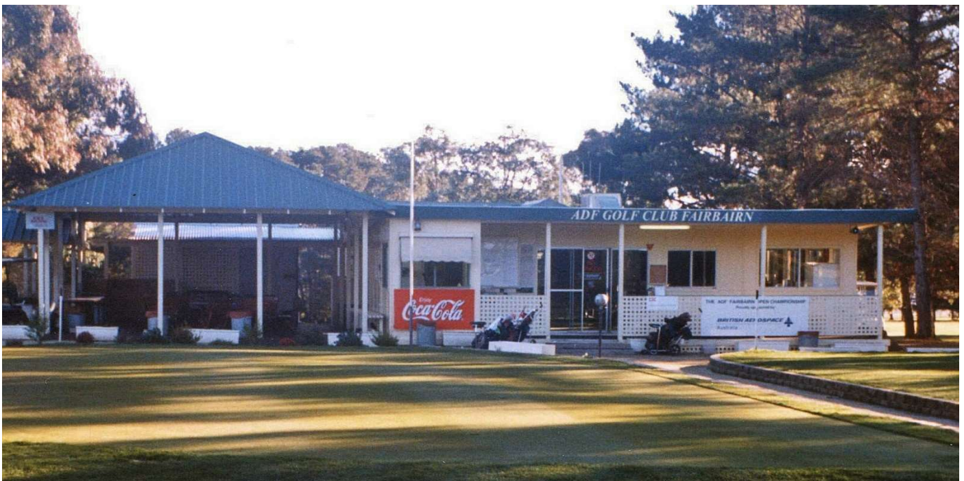
IMAGE H3 – the extended clubhouse (photo July 1999)
